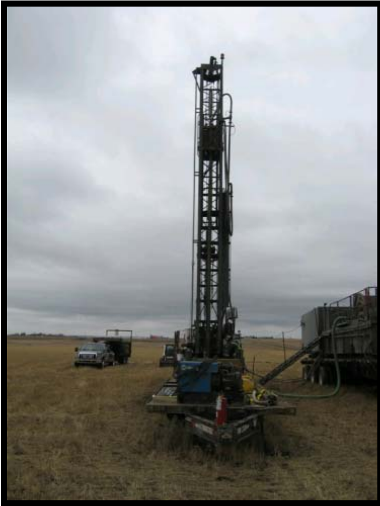
Images of the Drill rig set up
